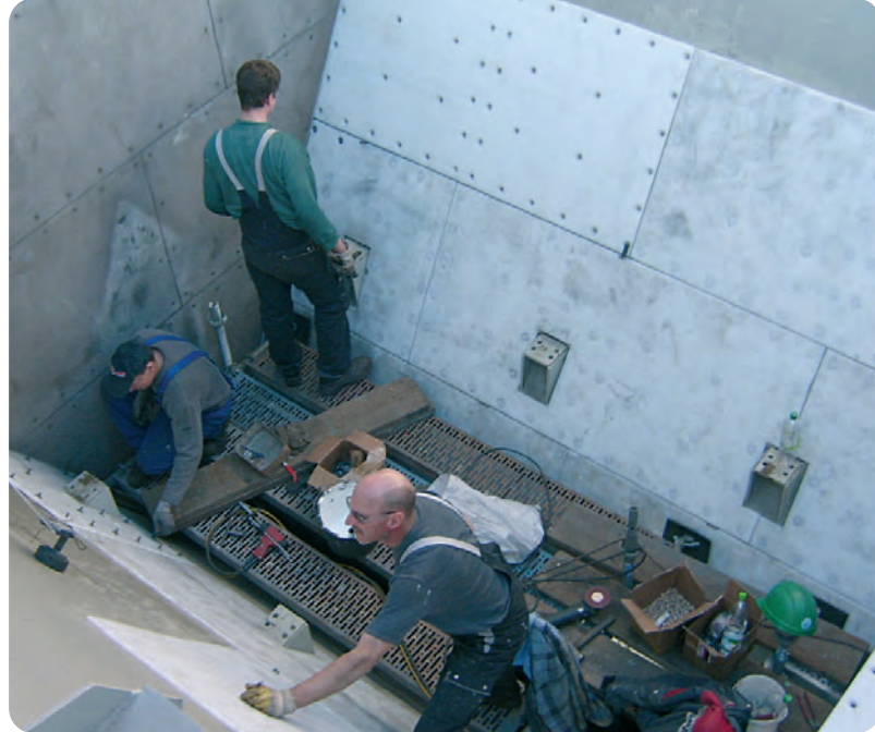
Stud-welding process: lining a hopper
