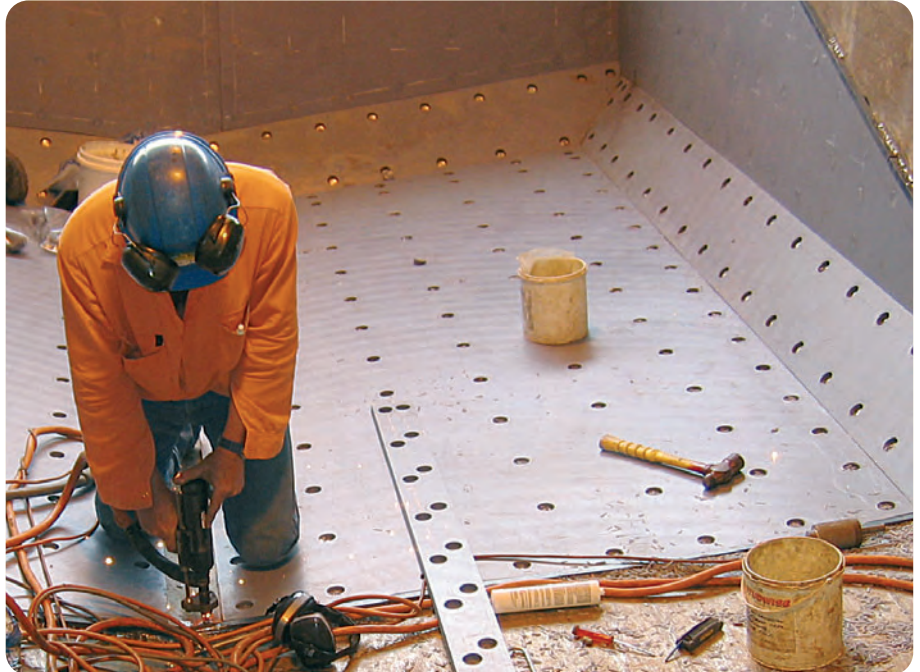
Expertise on site: Our experienced installation partners are at your service
