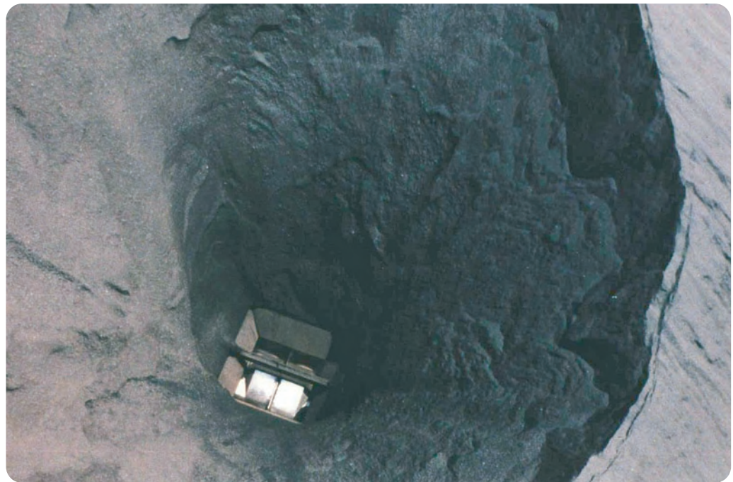
Rathole: The centre portion of the bin empties first in the form of a funnel (Photo Courtesy of Solids Handling Technologies, Inc.)
