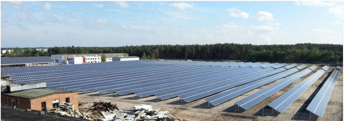
5.3MW Ground-mounted PV Plant in Arneburg, Germany
