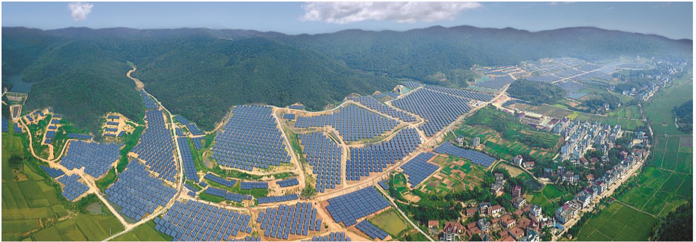
6MW Ground-mounted PV Plant in Exmouth, UK
