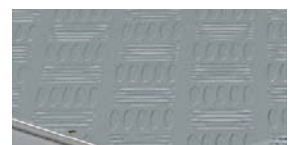
5 Structural metal plates to prevent slipping (on the largest box)
