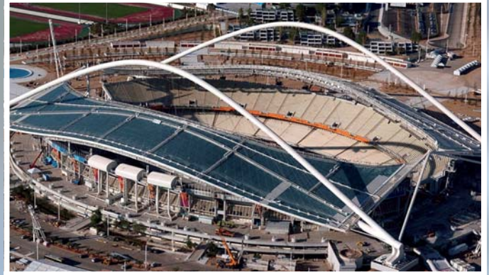
"Spiros Louise" Olympic Stadium, Athens, Greece (Roofing) 12mm PALGARD™ Solar Olympic abrasion resistant sheet & GA2004 System
