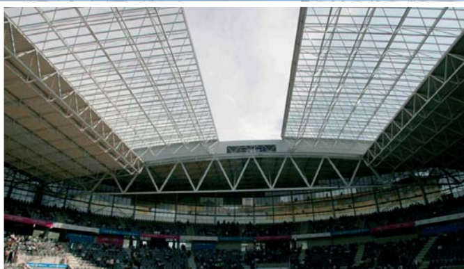
Plaza Del Toro Bullfighting Arena, Spain (Retractable Skylight) 10mm White Opal PALSUN® flat solid polycarbonate
