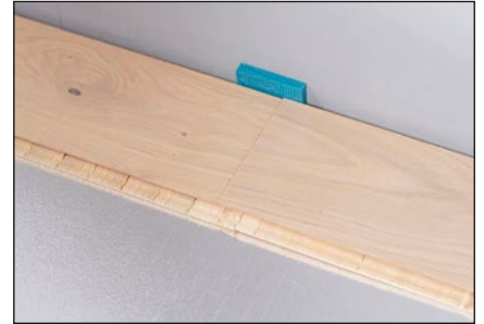
Use the plastic spacers to maintain a clearance of at least 10 to 15 mm from all walls and fixed objects in the room.
