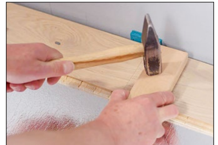
Join the end joints using a hammer and protective block. The long and end joints will connect automatically. Continue this installation process throughout the room.
