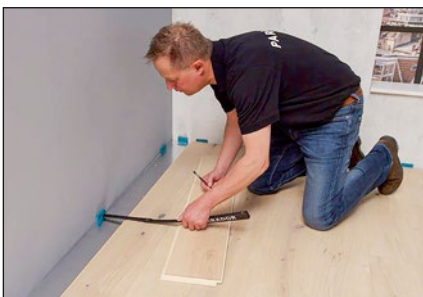
Use a leftover piece or the Parador MultiTool to transfer the wall outline to the last row of planks.
