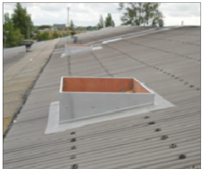
Example of base on sloping roof
