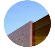
Bronze 80 C films are highly effective at reducing solar heat gain, whilst at the same time continuing to allow most natural light to pass through. They help reduce solar glare, conveying a touch of colour and customization to the external aspect of a building.
