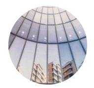
Alu 80 films are highly effective at reducing solar heat gain, whilst at the same time continuing to allow most natural light to pass through. Solar glare is greatly diminished and its one-way mirror aspect guarantees privacy from prying eyes, whilst affording a modern feel to the exterior of a building.
