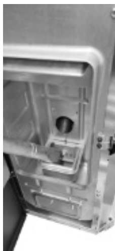
Fig. 35 - Burning pot box cleaning
