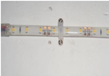
○ Installation is complete
