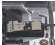
Drop cable splicing with fiber holder system
