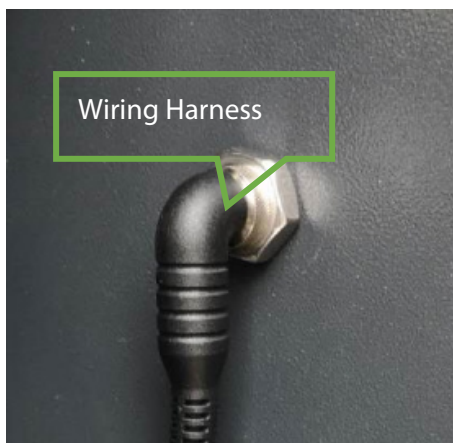
(c) Fix the radar inside the cabinet
