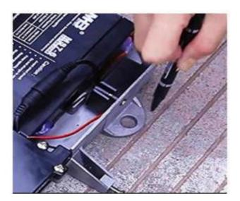
4. According to the position of the three mounting holes, with the model M12 drill bit, drill three diameter 12mm, 50mm deep hole, and knock the expansion bolt M8 into the hole, and then remove the nuts.
