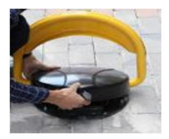
3. Use pen to mark the three holes to confirm drilling positions.
