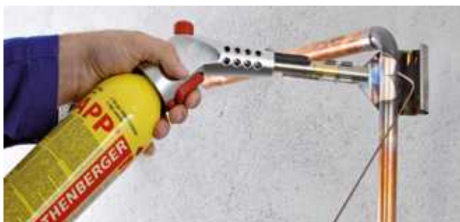
Brazing in gas installation
