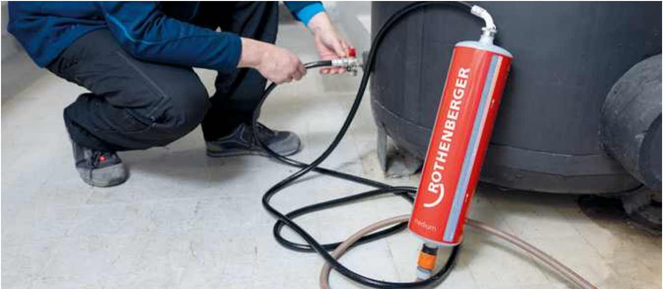
Filling heating systems according to standards
