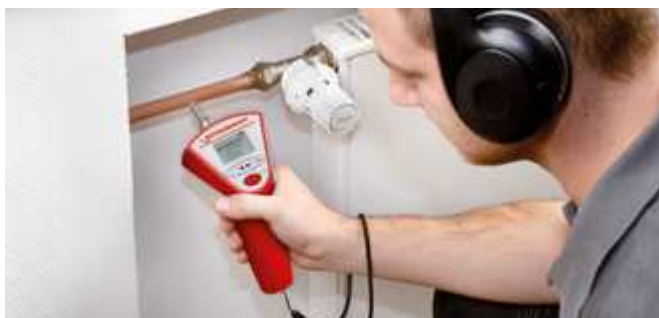
Acoustic leak detection of heating installations
