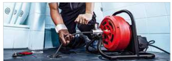
Cleaning of floor drain with 13 mm spiral
