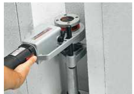
Work in confined spaces
