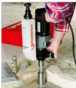
Drilling of the hardest materials
