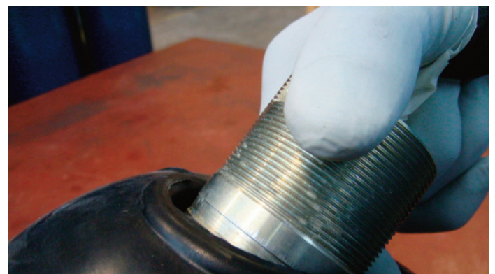
- Remove the gas valve, tilting slightly
