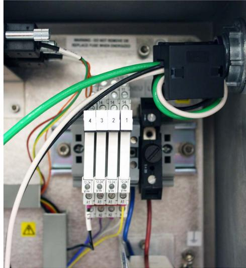
7. Strip back the jacket and/or insulation of the wires just enough to connect to the power terminal block.
