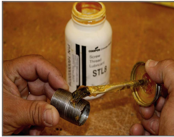
Figure 3-6 Applying conduit lubricant
