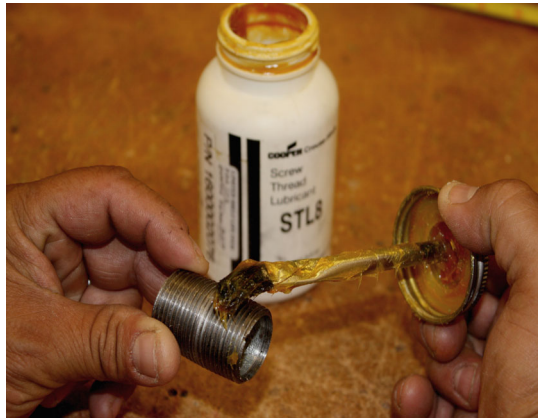
Figure 3-5 Applying conduit lubricant
