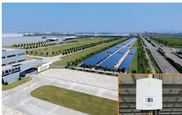
Shanghai Volkswagen Photovoltaic solar carport 55MW
