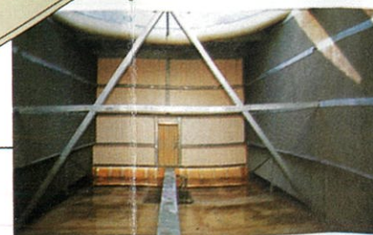
● Eliminator Preventing water splash made from PVC.
