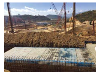
Dali East sea developing zone Utility tunnel
