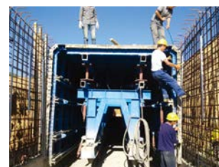
Dali East sea developing zone Utility tunnel
