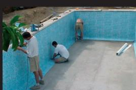
unrolled, horizontally, in one or more widths, according to the height of the vertical wall and allowing extra length of around 10 to 20 cm to enable the side panels to be welded to each other.
