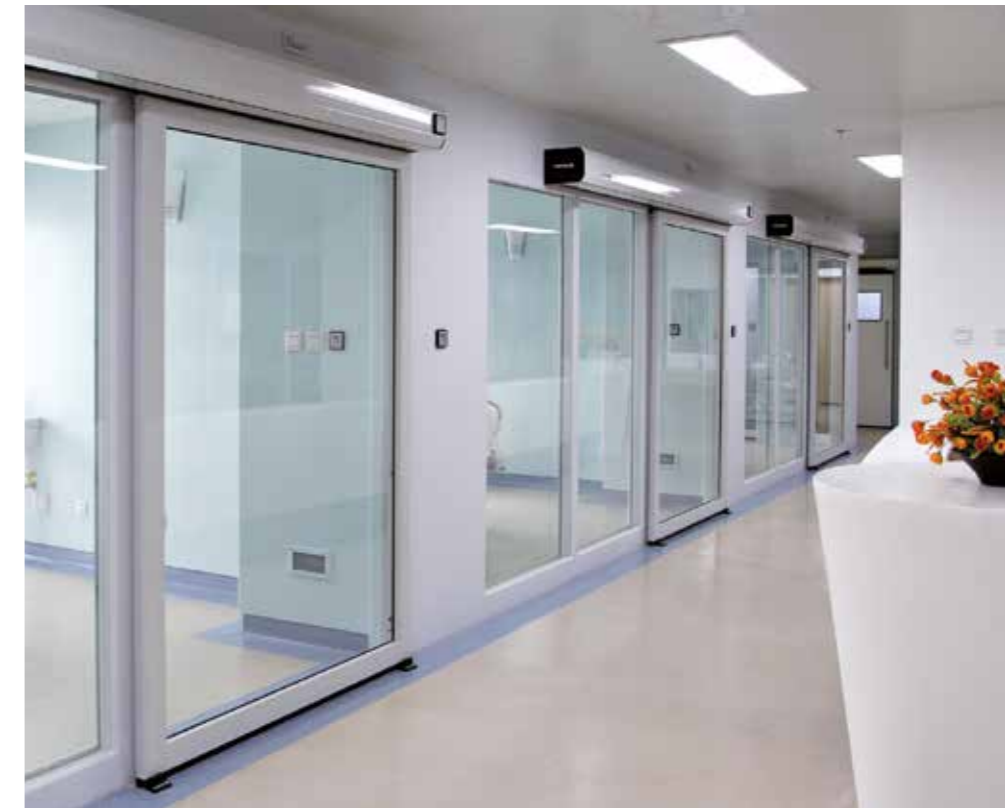
Clear View glass hermetic doors. Hospital ICU room.
