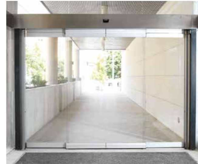
Panic break-out door without vertical stiles. Shopping centre.
