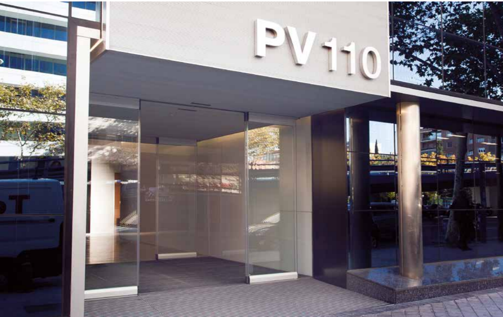
Panic break-out door without vertical stiles. Office building.
