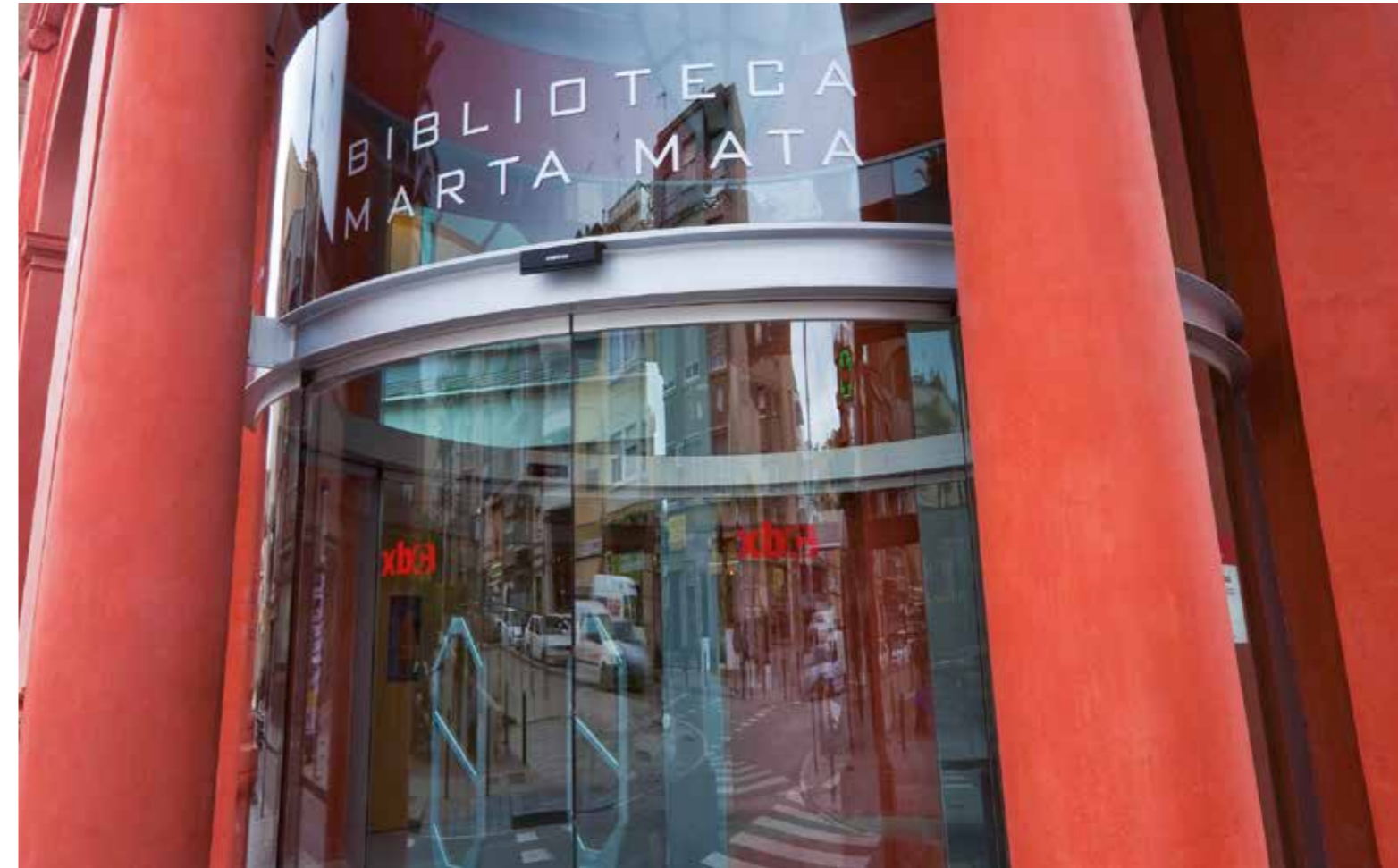
Circular automatic door. Library.
