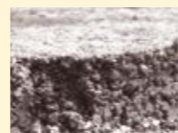
Roller compacted concrete
