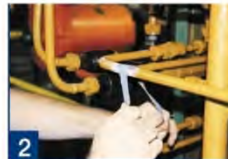
2 remove paint and clean pipe
