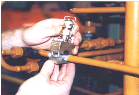
Installation on non-pressurized pipe Serv-Clip 2
