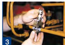
3 clamp SC onto pipe
