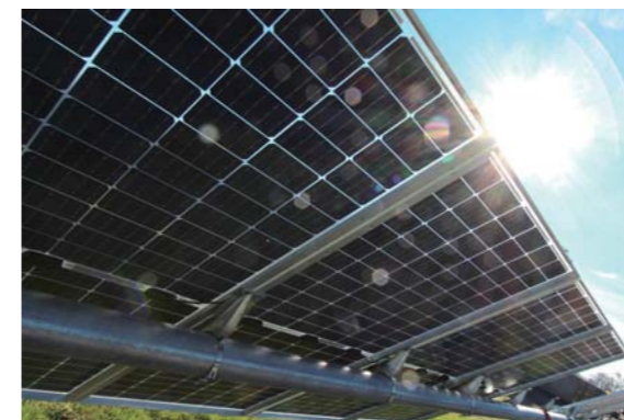
Bifacial module with transparent backsheet
