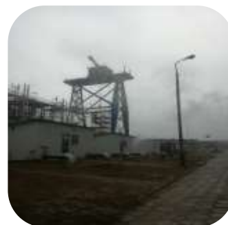
Large crane at fertiliser plant required a long term corrosion protection system. All surfaces were mechanically abraded and coated with 2 x coats of Resichem 55 Resinox
