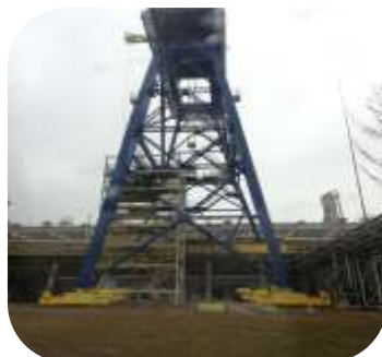
Large crane at fertiliser plant required a long term corrosion protection system. All surfaces were mechanically abraded and coated with 2 x coats of Resichem 55 Resinox
