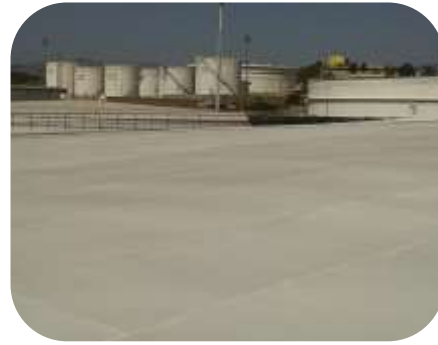
Crude oil storage tank roof was cleaned with high pressure water at 1000psi. Resichem 555 Resinox was applied in 2 coats at 500 microns wet film thickness per coat.
