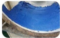
Coal grinder at a major European steel works was repaired using 204 Heavy Duty Ceramic Paste
