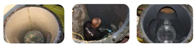
Sea water filter was in need of urgent repair. The internal surfaces were abrasive blast cleaned and lined with 2 coats of 202 Ceramic Repair Fluid. The coating was then post cured at 50C for 6 hrs to ensure the filter was back in operation within 24 hrs.
