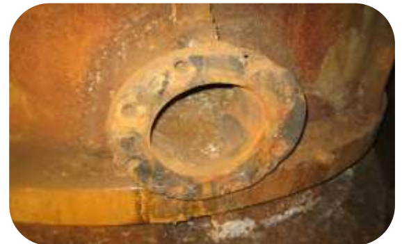
Damaged flange face repaired using 101 Metal Repair Paste
