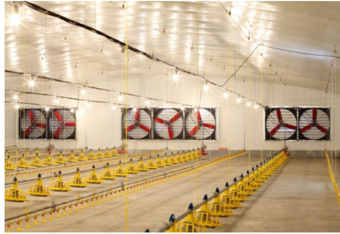
Poultry houses with Multifan fans in the Middle-East
