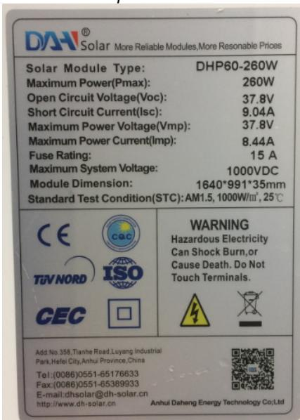
Fig. 23: Detail view of type label of
