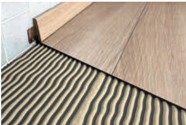
Full-surface glueing: Safe and permanent especially for commercial use
