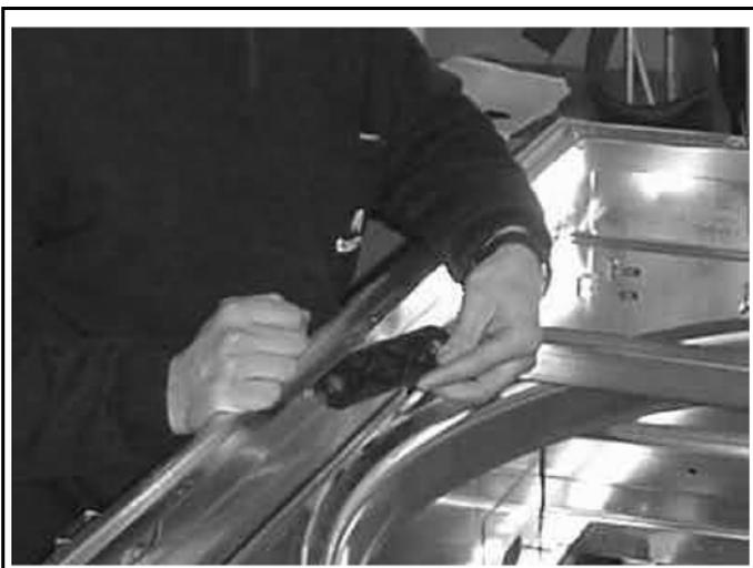
Place the oval plates between propeller central support and panels.
