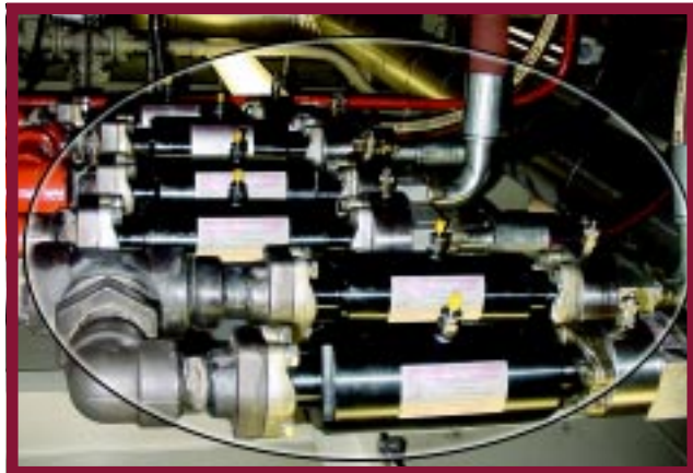
Due to space configuration, these six Suppressors were mounted in the lines leading from the pumps.
