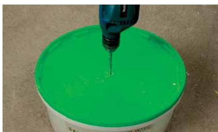
Drill a hole in the lid and mix the dry constituents with the lid on
