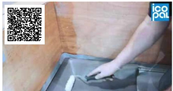
An open time of 5 to 50 minutes, based on drying conditions is recommended before assembly. Icopal TK 914 PVC Contact Adhesive must be allowed to dry until it does not string or stick to a dry finger touch.
