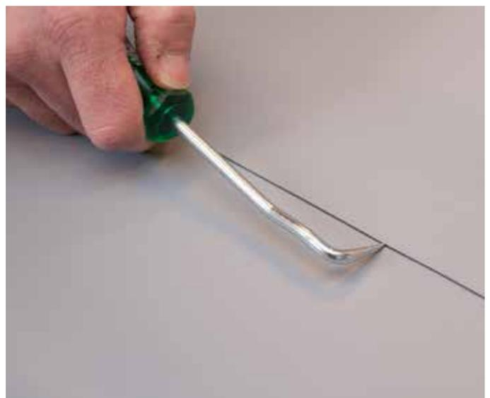
Always use a patch of 150 x 150 mm minimum with rounded edges. When the deficiencies are 'long', cut the patch to the size of the problem zone plus a 50 mm perimeter overlap. Circular patches shall have a minimum diameter of 150 mm.
