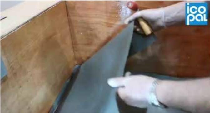
Roll the membrane onto the adhesive coated substrate while avoiding wrinkles. Immediately brush down the bonded portion of the sheet with a soft bristle push broom or a clean dry roller applicator to achieve maximum contact, without air pockets or wrinkles.
