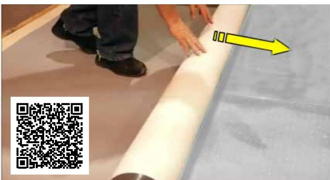
Once applied, roller the surface of the membrane using a weighted roller to encourage adhesion.
