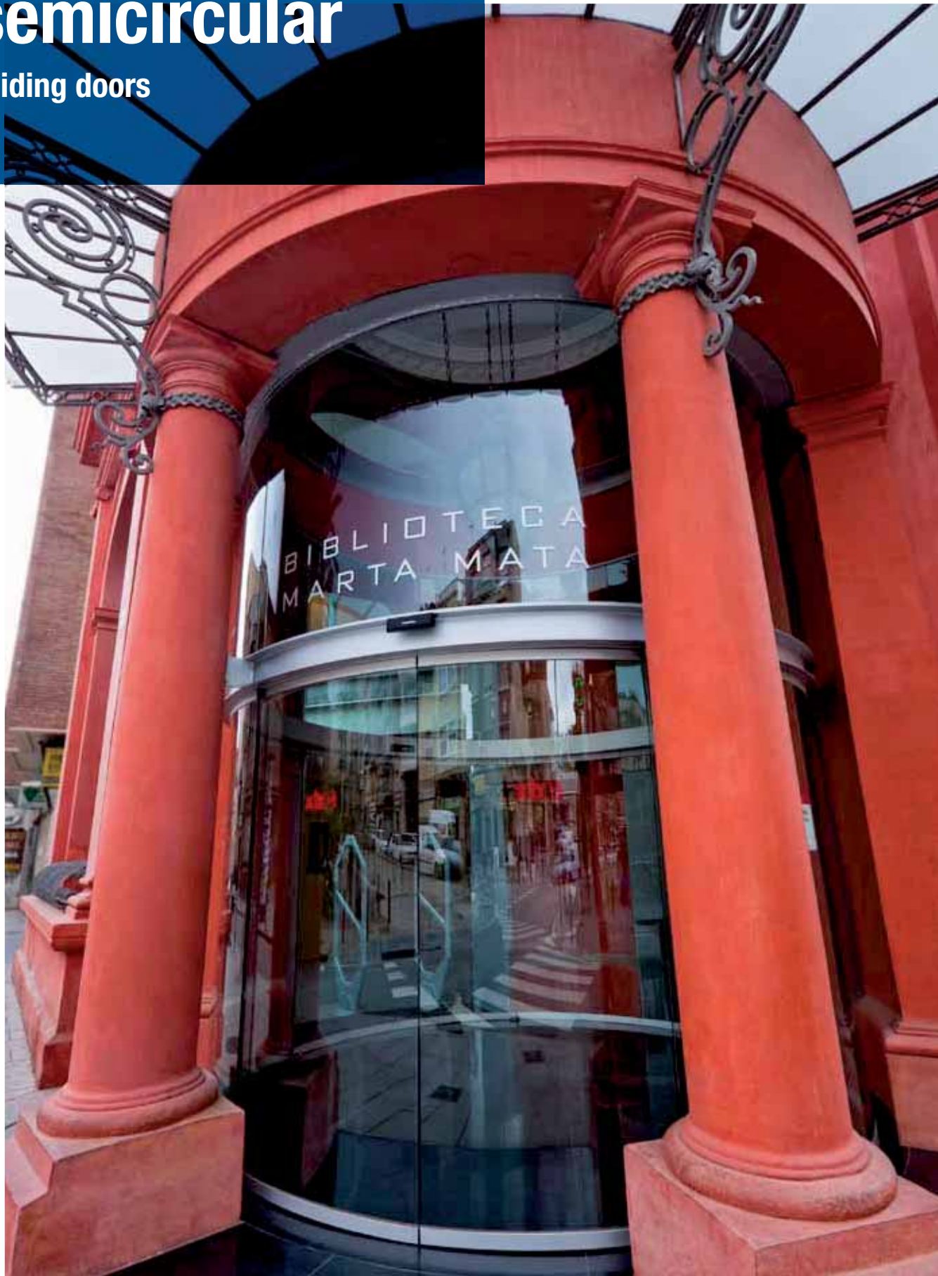
Circular automatic door. Library.
